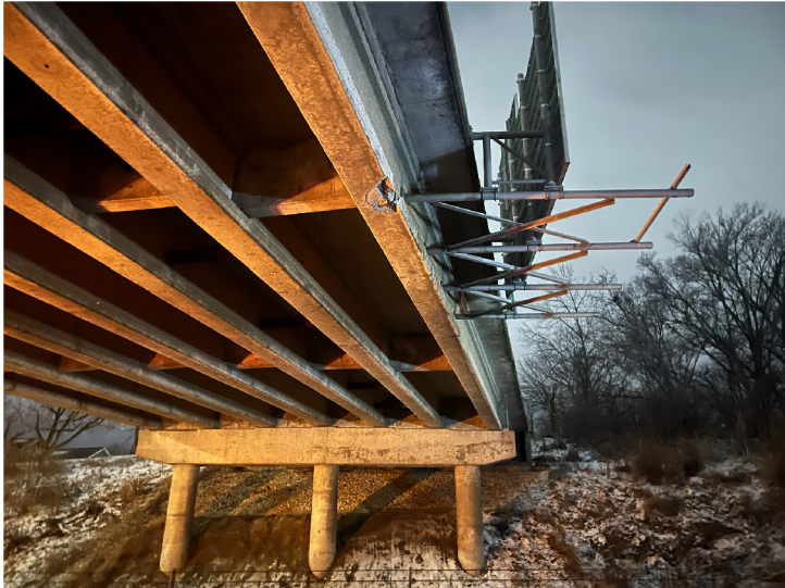
Span 2 Beam 1 Damage (Looking West)
