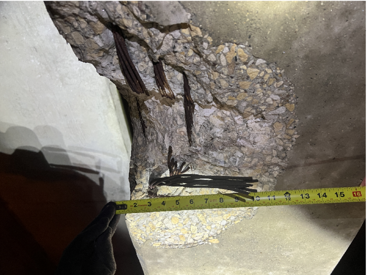
Span 2 Beam 6 Lower Face Damage (Looking Up)
