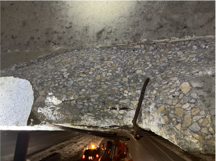
Span 2 Beam 1 Upper Face Damage (Looking South)
