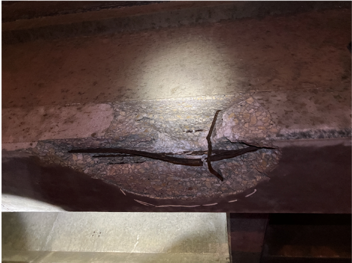
Span 2 Beam 1 Damage (Looking South)
