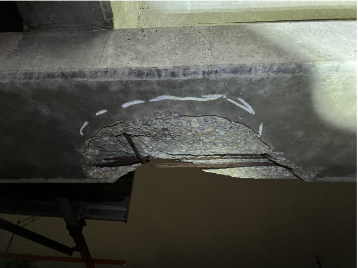
Span 2 Beam 1 Lower Face Damage (Looking Up)
